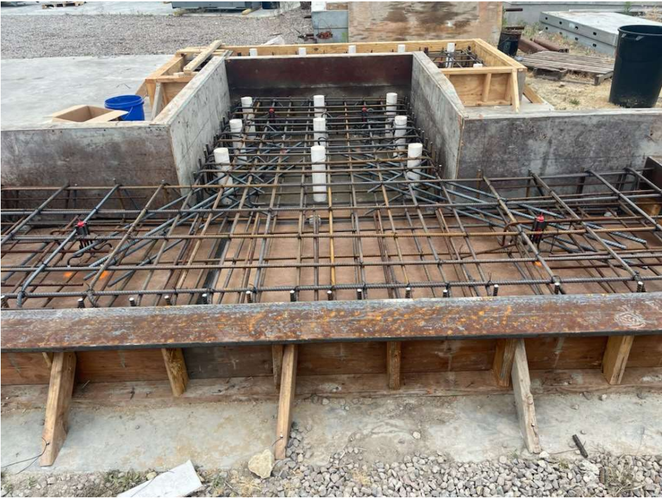
Foundation needed for expanding shake table
