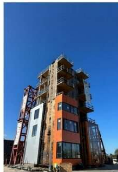
NHERI Converging Design 6-story Building Specimen
