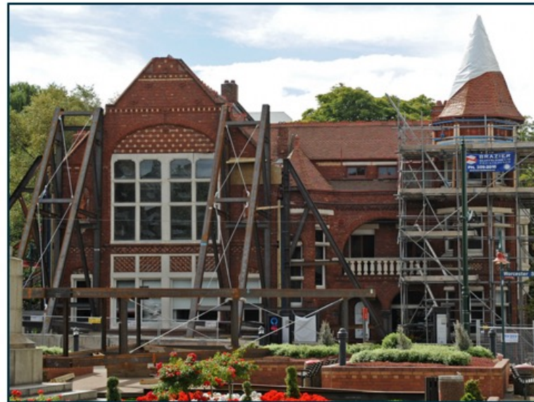
Masonry building retrofit
