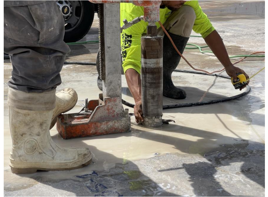
Concrete core collected from the basement slab
