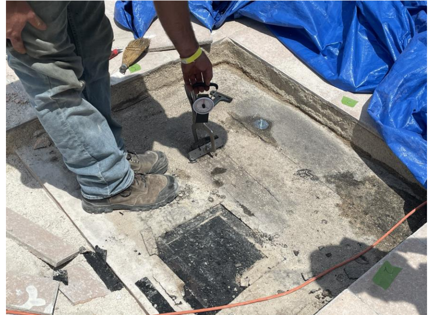
Waterproofing testing at the pool deck
