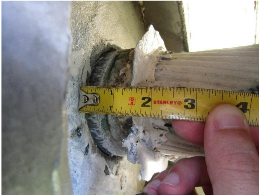
A12W AUX showing about 1 3/8-inch extension (May 2018)
