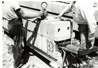
Prestressing of masonry beams
