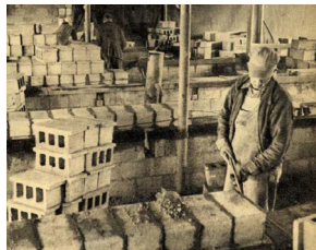
Blocks being mortared
