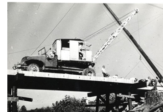
Prestressed masonry beams lifted into place
