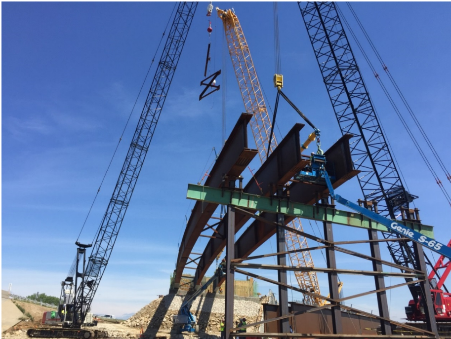
Gateway Interchange Flyovers, Johnson County, KS
