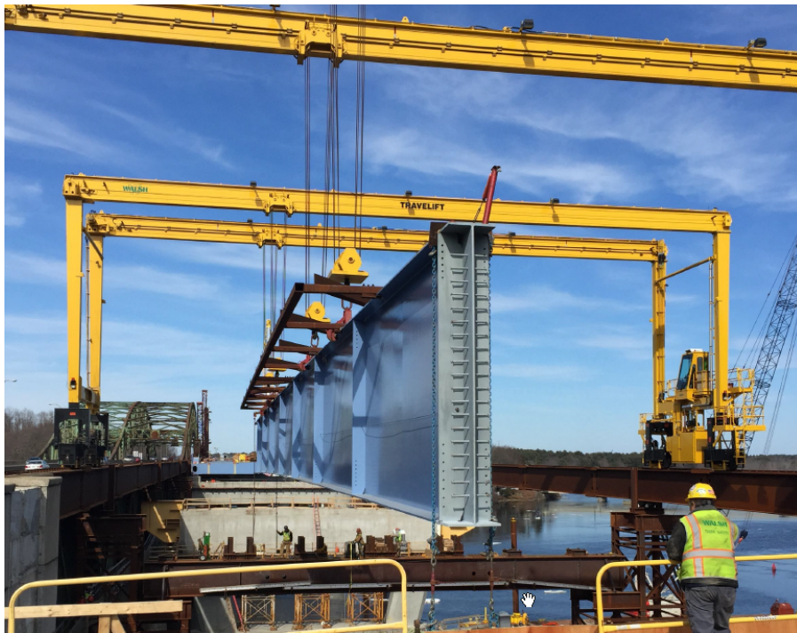
Whittier Memorial Bridge, Newburyport and Amesbury, MA
