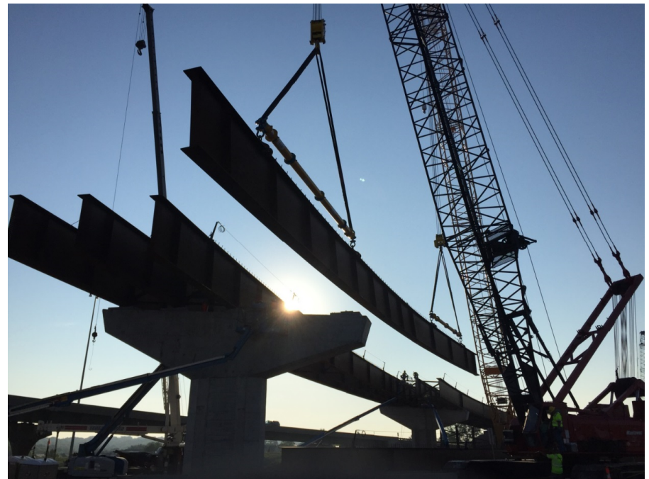
Gateway Interchange Flyovers, Johnson County, KS
