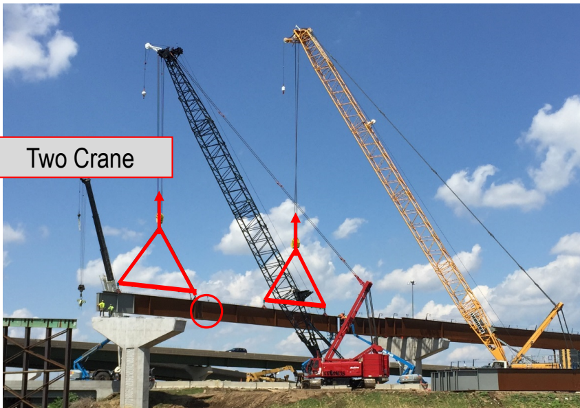
Gateway Interchange Flyovers, Johnson County, KS
