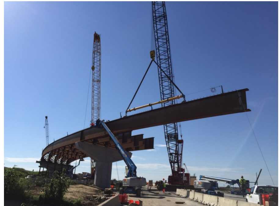
Gateway Interchange Flyovers, Johnson County, KS
