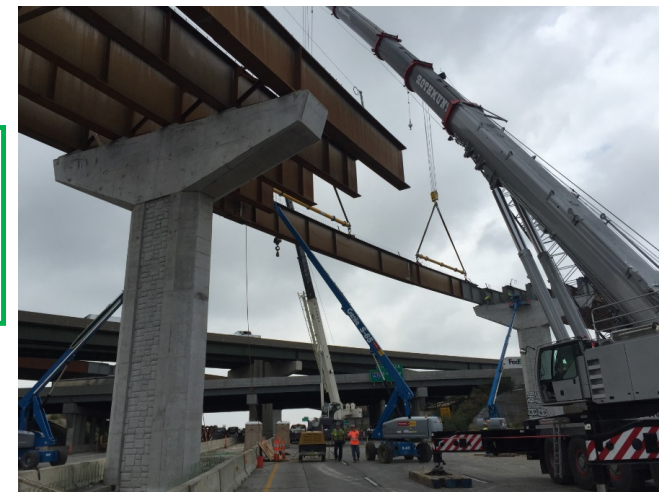
Gateway Interchange Flyovers, Johnson County, KS
