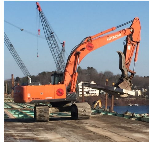
Sarah Long Demolition, Portsmouth, NH
