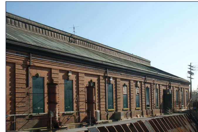
1889 - New Orleans Structural strengthening
