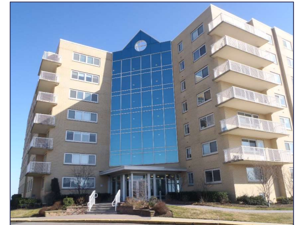
1963 - New Jersey coast "Architectural" maintenance
