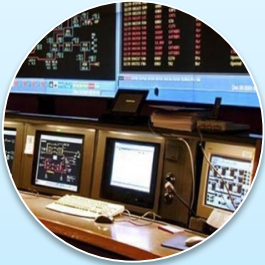
Advanced Distribution Management System (ADMS)
