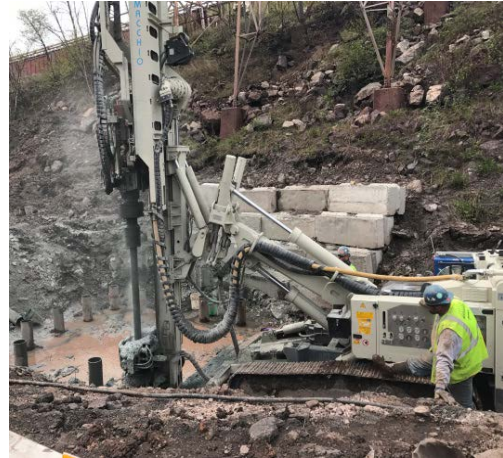
Fig. 5 – Micropile Drill Rig
