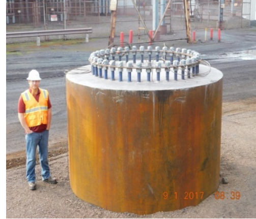
Fig. 4 – Foundation at STR 617
